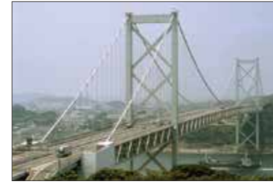
The bridge connecting Kyushu to Honshu
